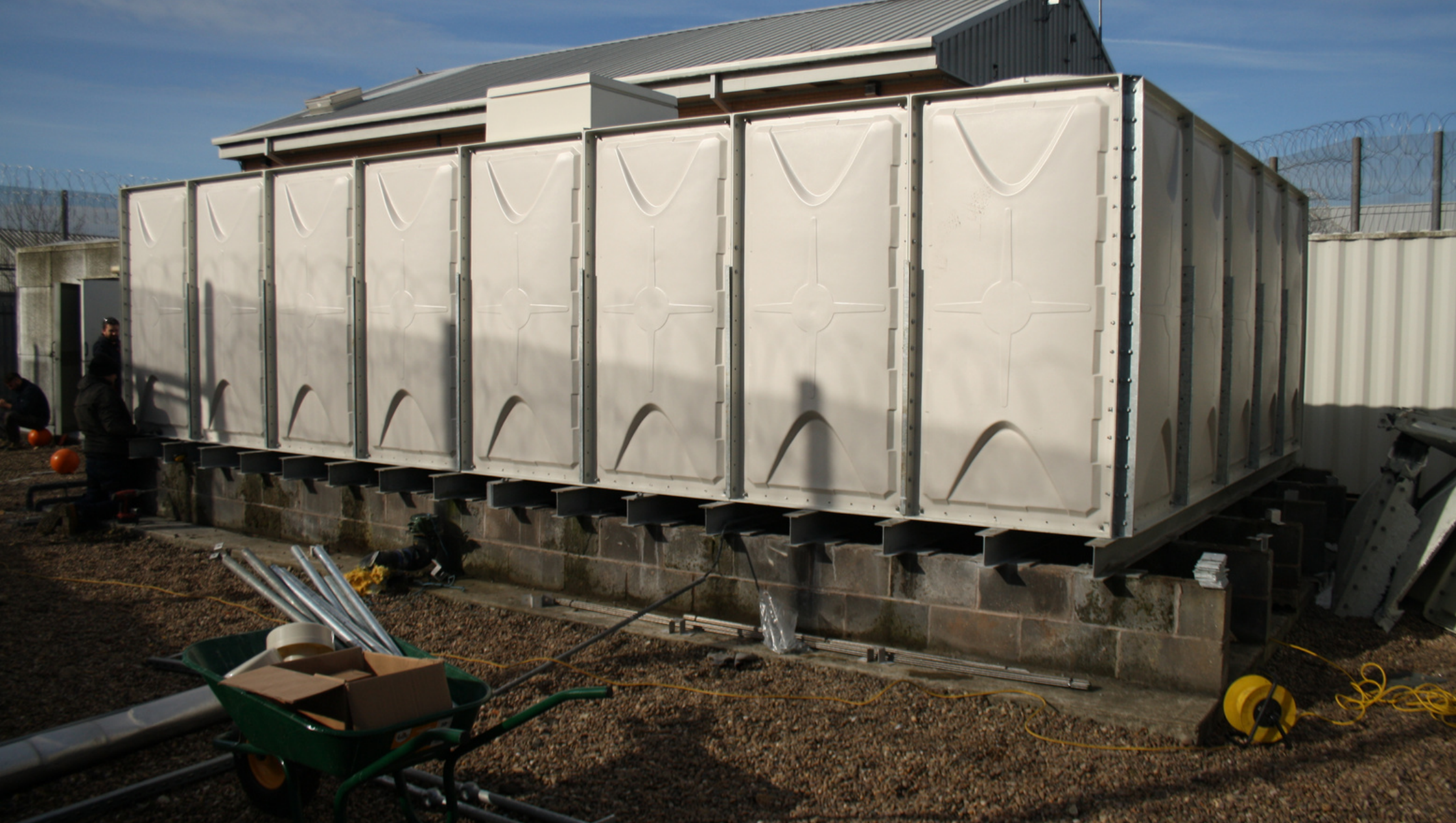
AN EXAMPLE OF A 8X5X2 METRE GRP WATER TANK REPLACEMENT CARRIED OUT AT A SECURE FACILITY IN THE UK
